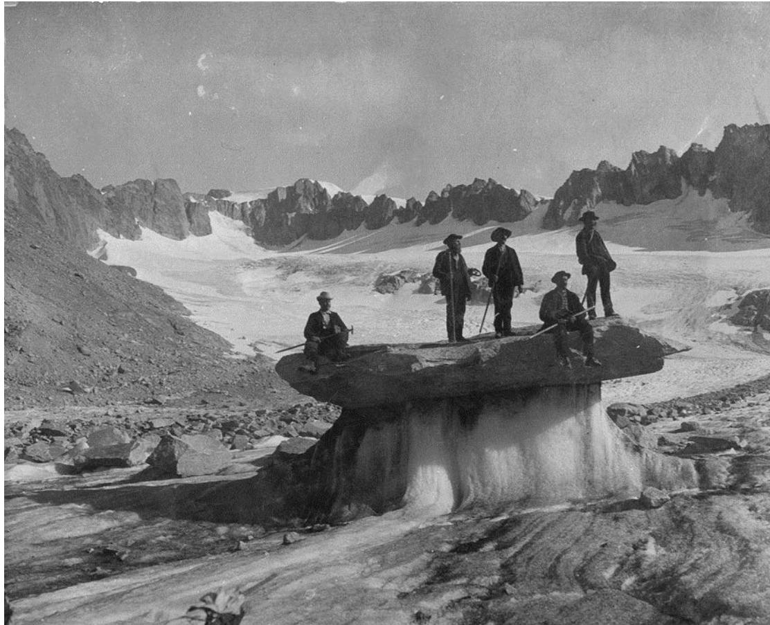
Topographer II. Class Heinrich Wild (left) around 1902 on a boulder in the Rhone glacier. He observes, measures and documents its development with Leonz Held and Max Rosenmund. It is the first geodetic study of glacier movements. ((SK KF 15/16)).
