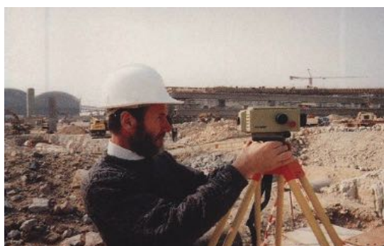
Construction of Hong Kong's Lap-Chek-Kok Airport in 1996 with the Wild DNA2000 digital level.
